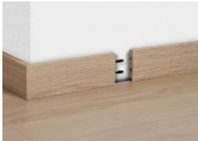
Connection of 2 skirting boards along the wall
